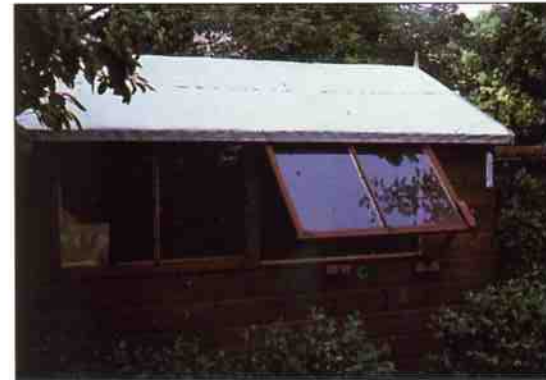
Fig. 2. Painting the roof white can help reduce thermal gain in a partially shaded shed. As well as the door, the window is left permanently open and the space covered with chicken wire.
